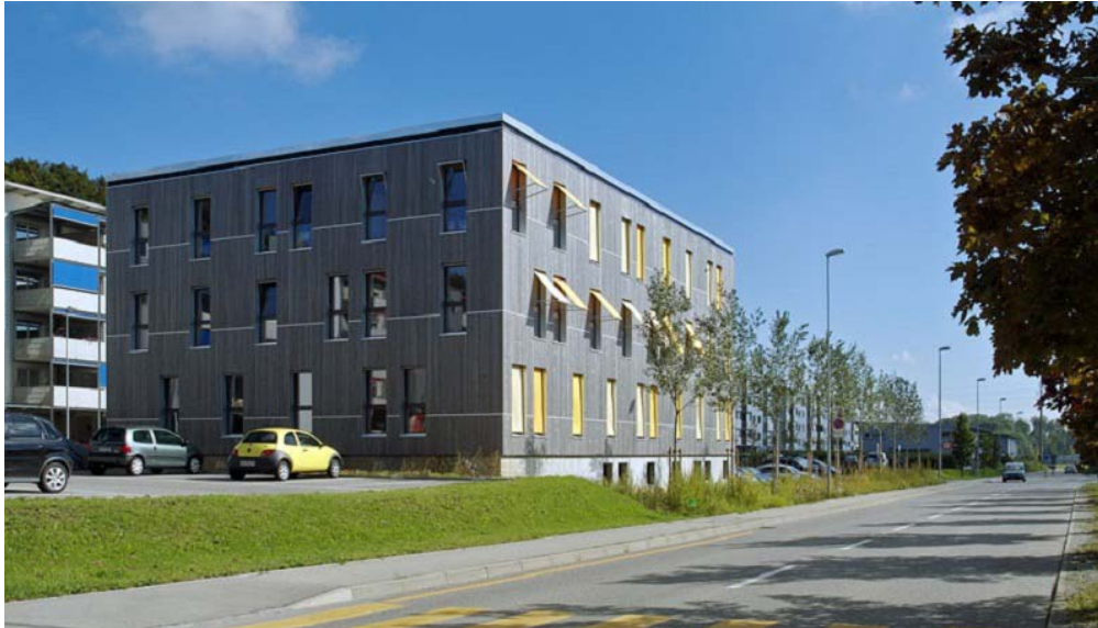
Figure 10: Green Offices Givisez, Switzerland
